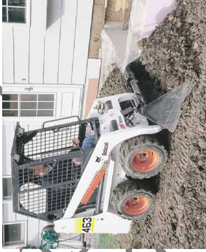
DOT / Cal-Trans Approved Class 2 Crushed Aggregate Road Base Mat'1 Installed with "Bobcat" Mini-Tractor When Accessible
